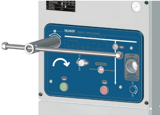
Insert the lever into spring charge lever hole and rotate in the direction of arrow. **(Clockwise)**
